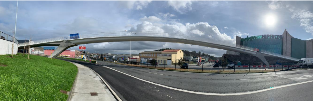
Fig. 14. Final appearance of the footbridge
