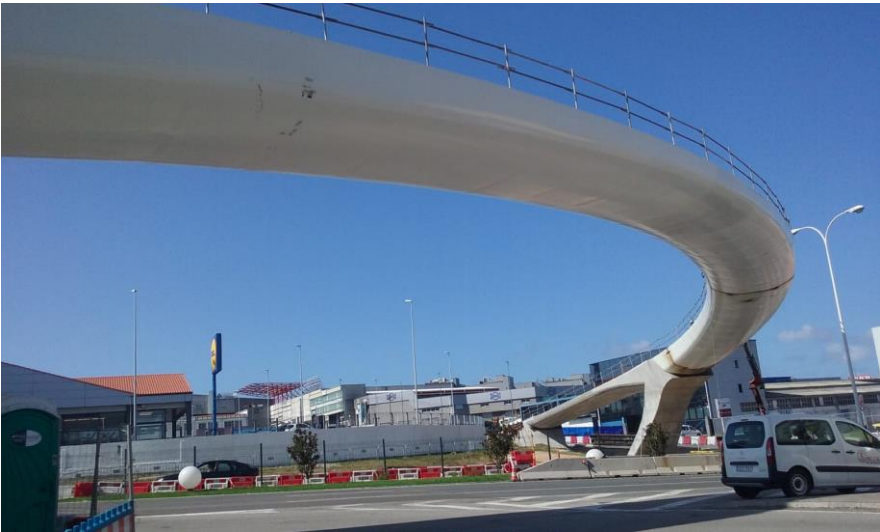
Fig. 13. Temporary support at midspan removed
