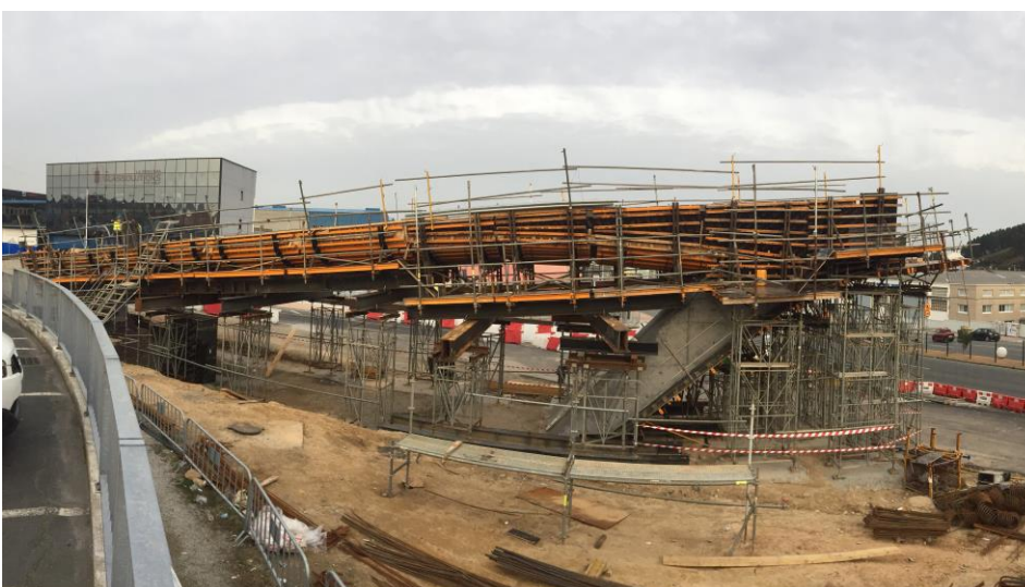
Fig. 9. Scaffolding system for lateral spans
