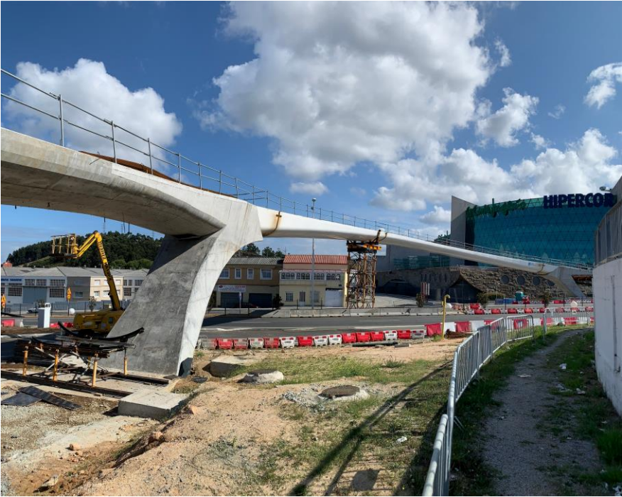
Fig. 12. Steel deck finished with temporary support at midspan
