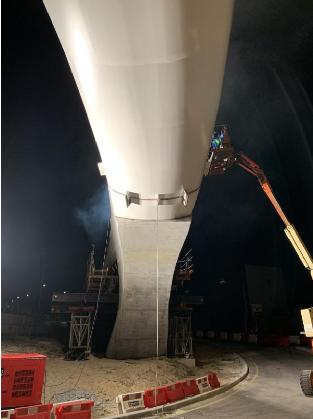
Fig. 10. Erection of the first steel segment of the deck
